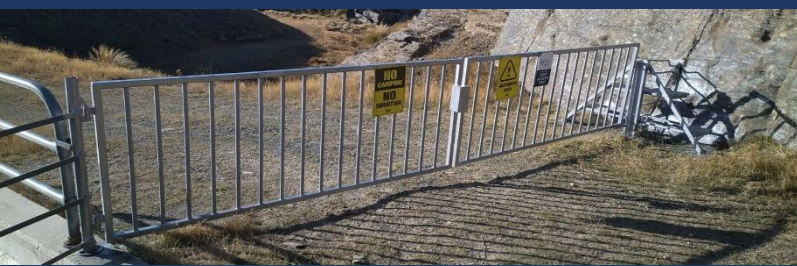
Image: New Loganburn Dam Wall restricted vehicle access gate, with foot access stile for fishermen at far end.
