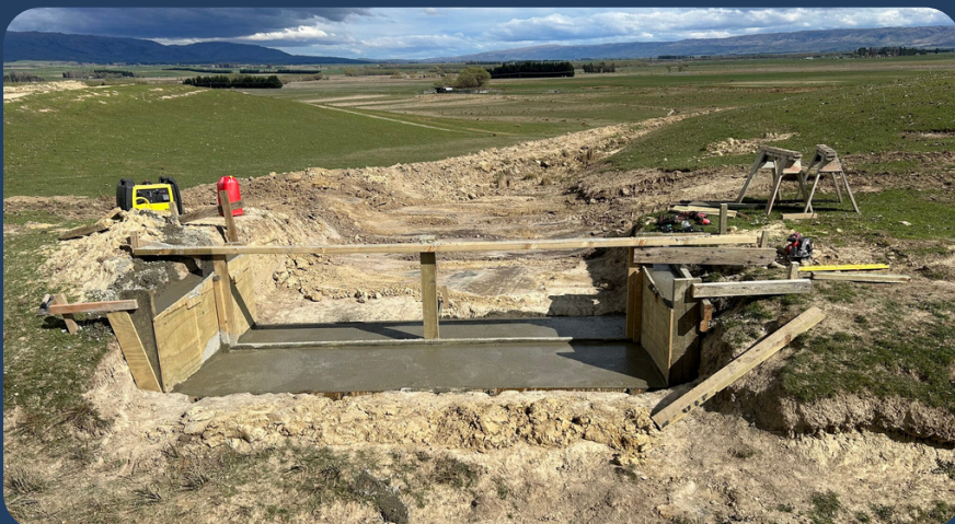
Overflow Weir for better control - being built by Brent
