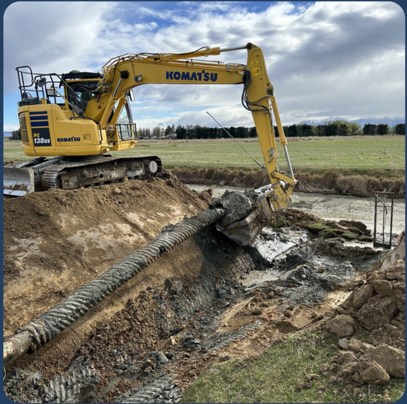
Redundant Take Removal & Race Repair
