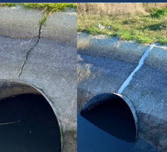
Photo: Repairs by Alastair at the Waipiata Gate Siphon with a PF rod and Hume Bond
