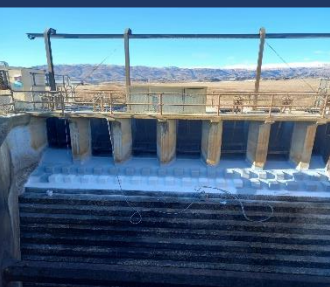
Photo: Epoxy coating on stairs below Linnburn Gates – Main gates to the Westside and Waipiata Scheme
